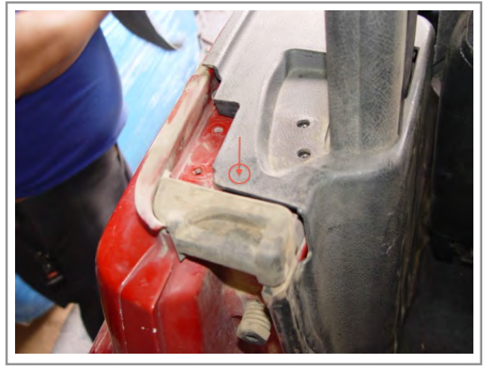
8. Drill a 3/4" hole in the plastic or cut a section out, to expose the bolt hole from step 6.
